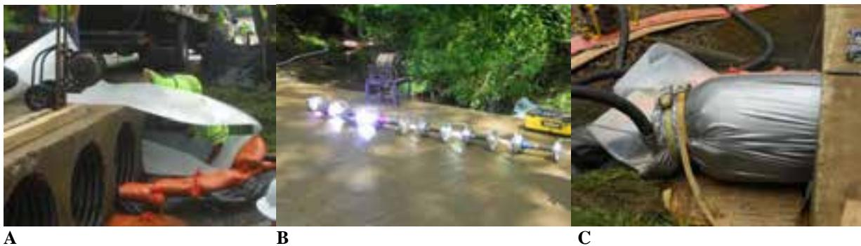
**Figure 3. A: Installation of UV CIPP Liner, Illustrating Slipsheet Insertion; B: UV Light Train Prior to Insertion in Liner; C: Liner Inflation During UV Cure.**
