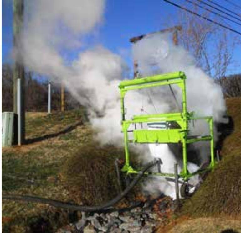
**Figure 2. Curing Process During Vinyl Ester Based CIPP Installation**
